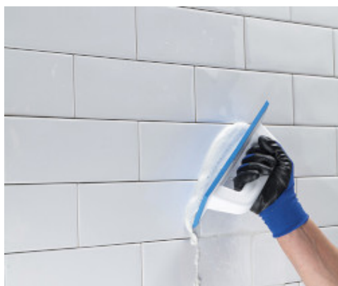
Application of Keracolor SF with MAPEI trowel
